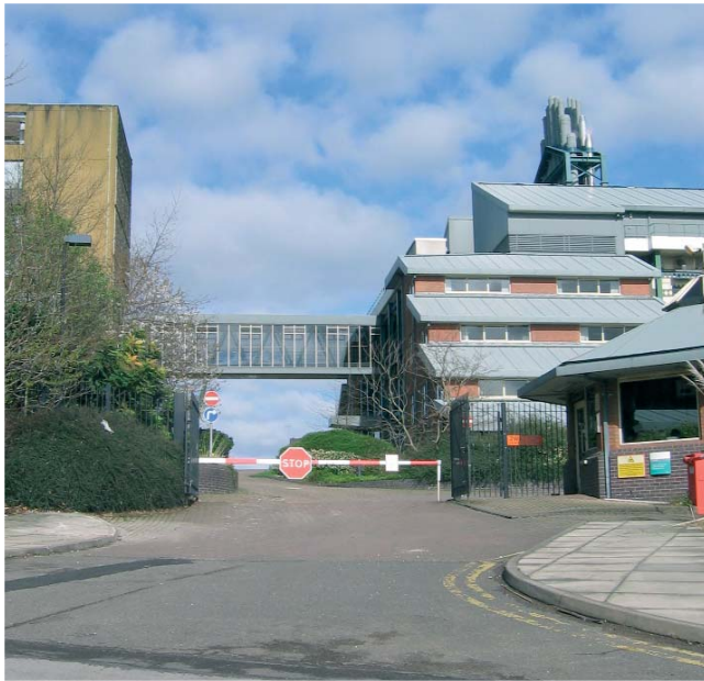
RE-OPENING THE PRIVATISED STREET THROUGH THE HSE SITE IS A PRIORITY
