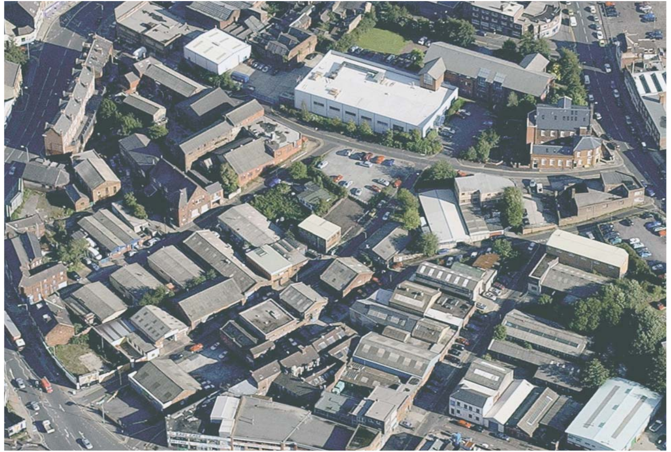
AERIAL VIEW OF FURNACE HILL
