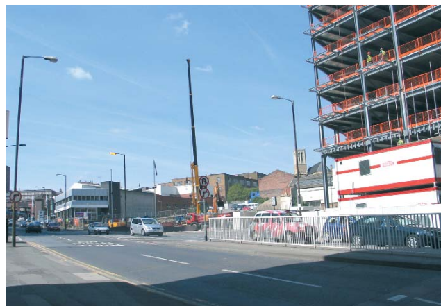
TENTER STREET AT PRESENT
