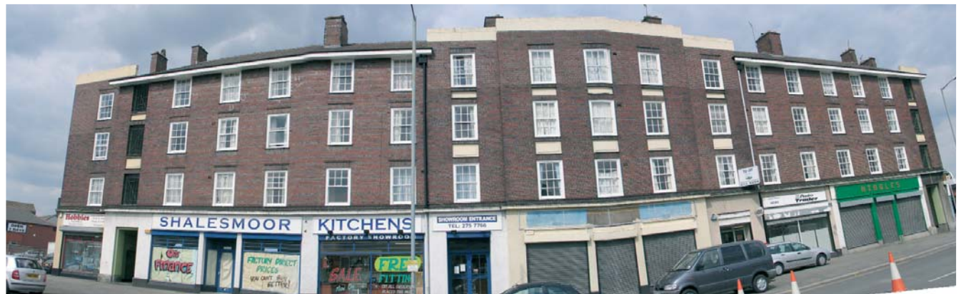
MOORFIELD FLATS, SHALESMOOR TO BE RETAINED FOR SOCIAL HOUSING
