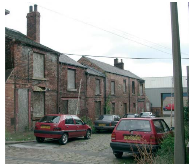
AS EXISTING - VIEW NORTH-EAST ALONG WELL MEADOW STREET
