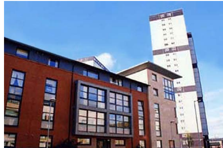
Modern apartments in Brown field "social housing" context
