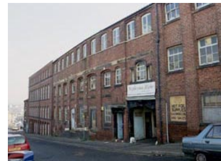
Upper Allen Street C19th works
