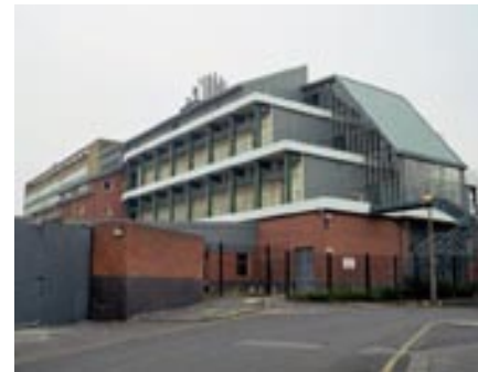
Health & Safety Complex
