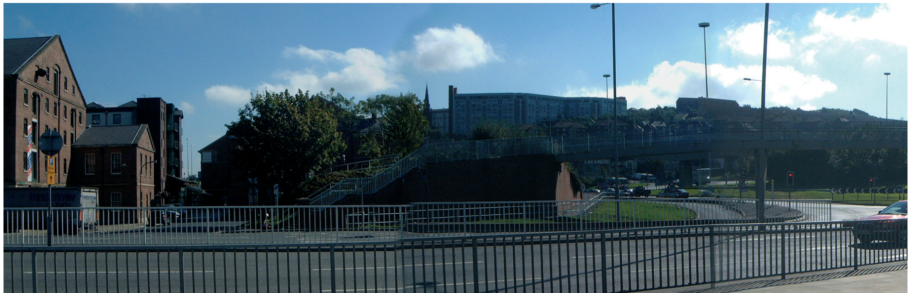
Exchange Place looking onto Park Square
