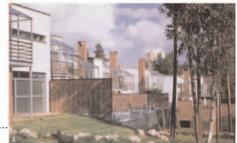
Cascading terrace, using brick
