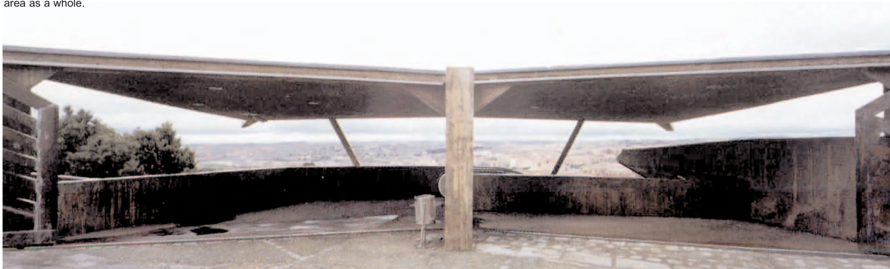
Dramatic shelter framing view of city centre
