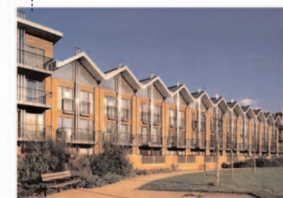
Housing fronting on to the park, dense but light, with large areas of glazing
