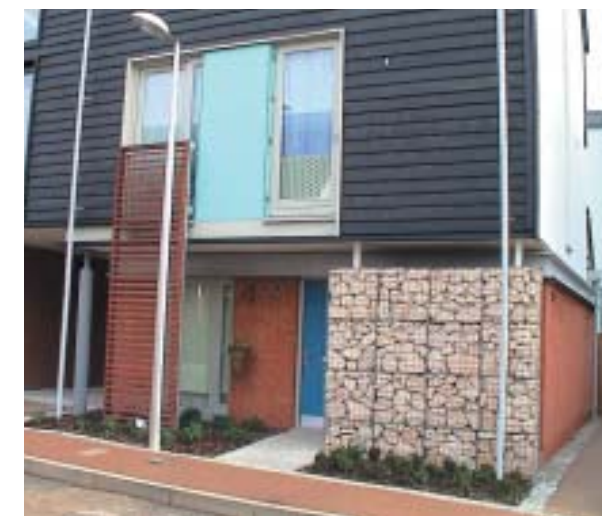
21. Housing quality New Hall, Harlow
