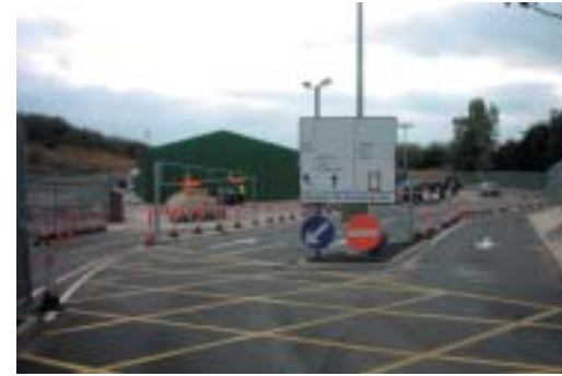
14. Waste Disposal Compound
