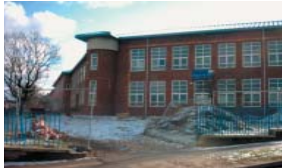
1. Herries School building entrance Penrith Road
