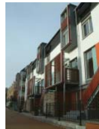
16. Strong housing frontages creating distinctive streets (Newhall, Harlow).
