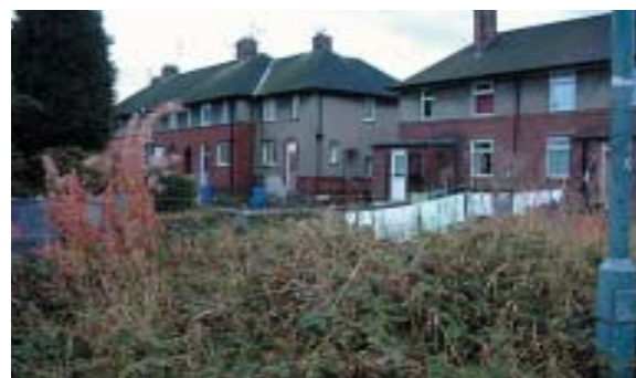
10. Houses back onto Parson Cross Park, with security risks
