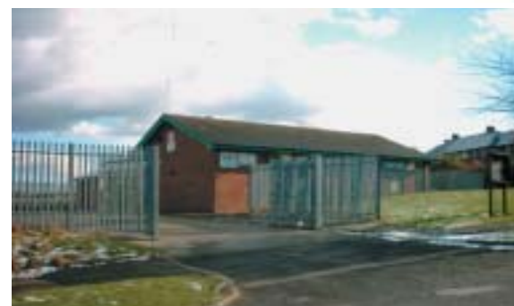
9. Adlington Community Centre: unrelated to its surroundings and the community
