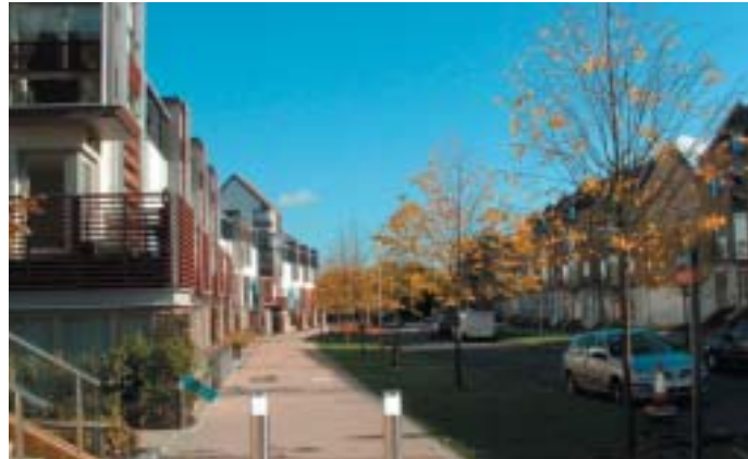
16. Example of a main residential street (Newhall, Harlow) illustrated in Fig 13
