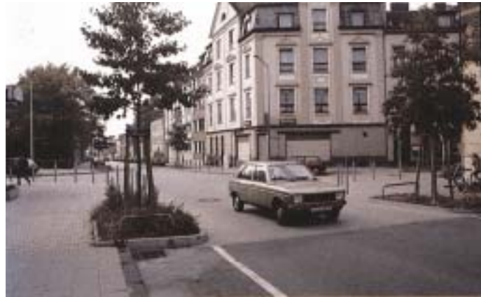
15. Example of street treatments at key intersections (Aachen, Germany) illustrated in Fig 15
