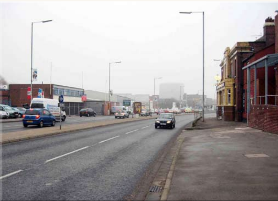
Photograph 19. The large Neepsend Gas Holder dominates the long views along the dual carriageway when looking towards the city centre.
