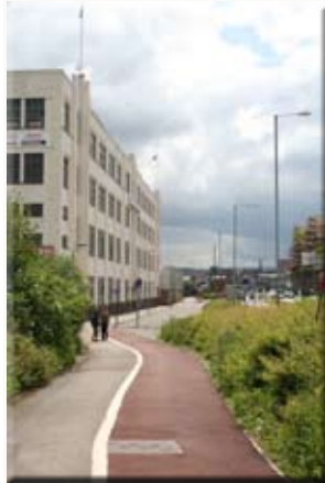
Photograph 20. The large, white former Hydra Tools building to the left, viewed looking towards the city centre from the north.
