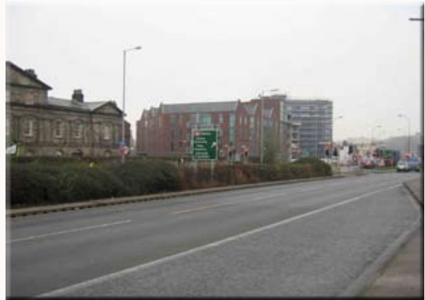
Photograph 21. Recently constructed apartment blocks dominate the view looking towards Kelham Island alongside listed buildings such as Globe Works.
