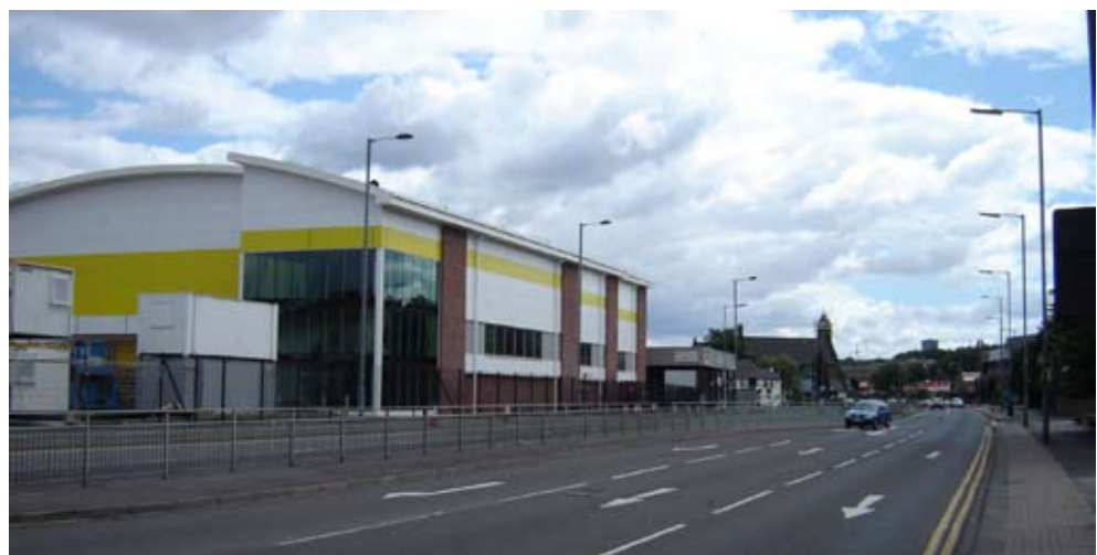
Photograph 23. Big Yellow Warehouse, with a green roof on Penistone Road
