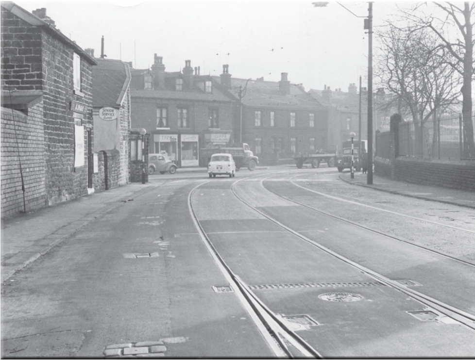
1960's Photograph 3. Parkside Road looking towards Penistone Road. The terraced houses fronting Penistone Road were demolished during the widening of the A61.
