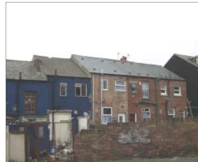
Exposed boundary walls on Brotherton Street
