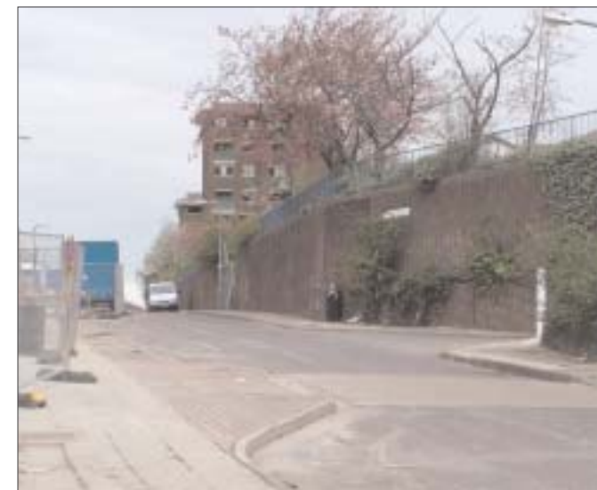
Tall retaining wall along Pye Bank Road
