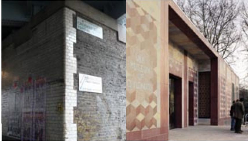
The improvement of facades and entrances to existing community facilities will improve the most public buildings in Flower, Brushes, Stubbin and Firth Park
