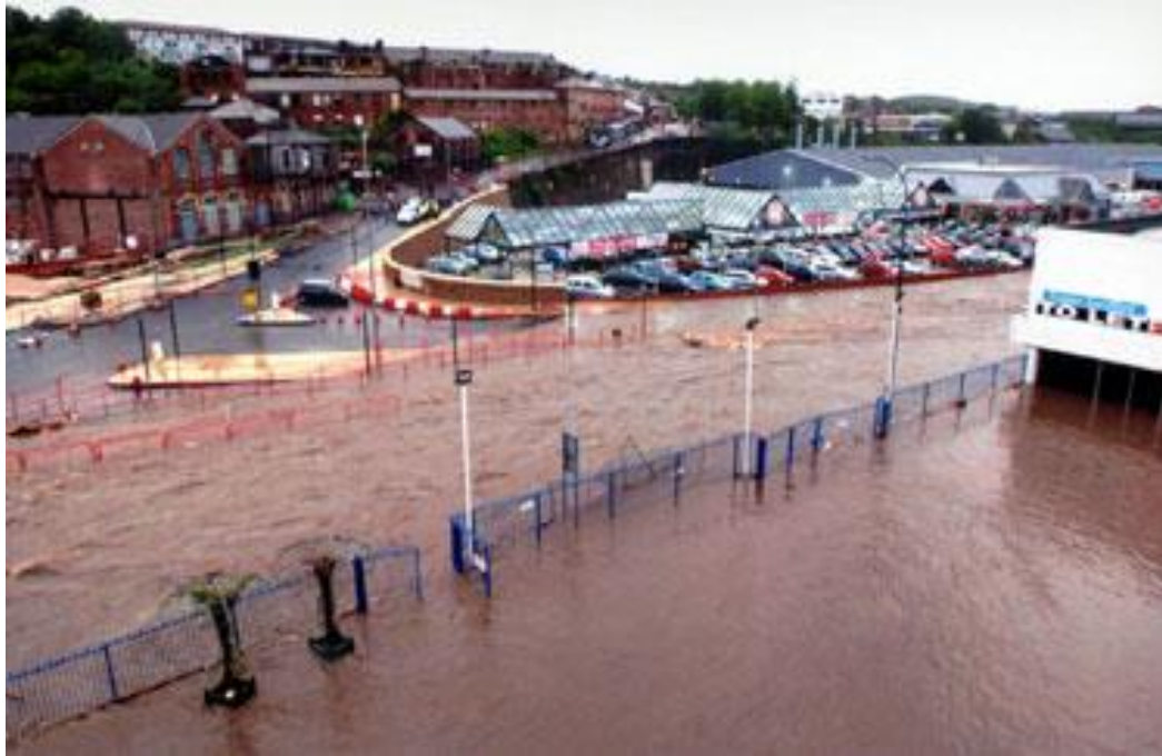
Saville Street looking towards Spital Hill after flooding caused by heavy rainfall 2007 ( Sheffield Local Studies Library: Picture Sheffield u04445 )
