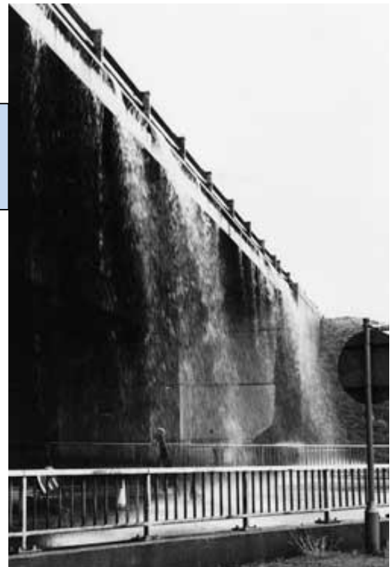
Water pouring off the M1 Tinsley Viaduct onto Sheffield Road, during flood event in May 1979 ( Sheffield Local Studies Library: Picture Sheffield s26926 )
