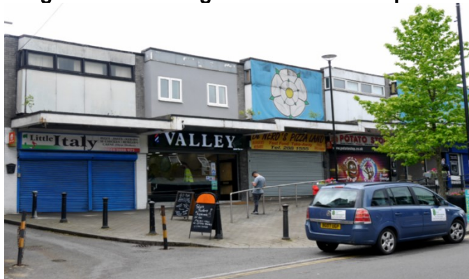
Image 1: Stocksbridge Towns Fund Shop Fronts Current
