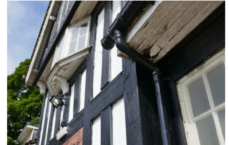
Photo of rear rainwater gutter and roof fascia / soffit detail showing major deterioration in timber panelling, due to missing and cracked roof tiles. Also showing evidence of bird nesting.
