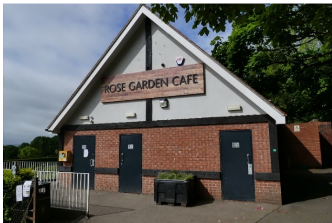
Photo of east facing side elevation of the new WC block to the Rose Garden Café.
