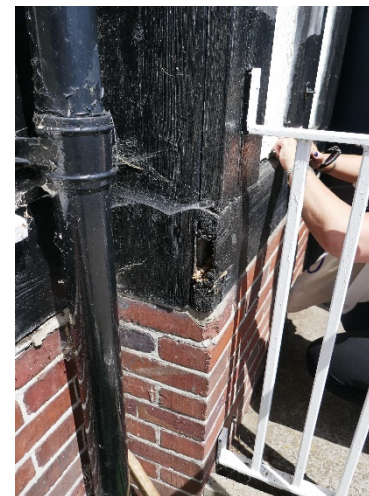
Photo of front elevation showing deterioration and cracking in timber and render façade.
