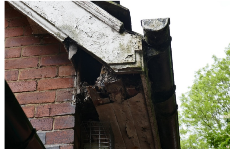
Photo of rear rainwater gutter and roof fascia / soffit detail showing major deterioration in timber panelling, due to missing and cracked roof tiles. Also showing evidence of bird nesting.
