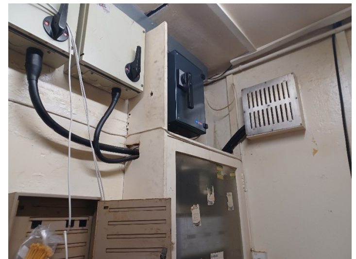
Photo showing existing electrical installation mains units and incoming supply
