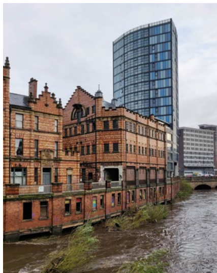
Royal Exchange Buildings, The Wicker
