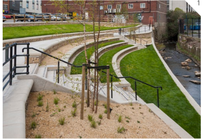
Matilda Street- Example of a riverside park which interacts with the waterside edge by terracing towards the water, creating attractive seating areas and opportunity for greenery and vegetation. A path along the edge clearly defines the pedestrian route
