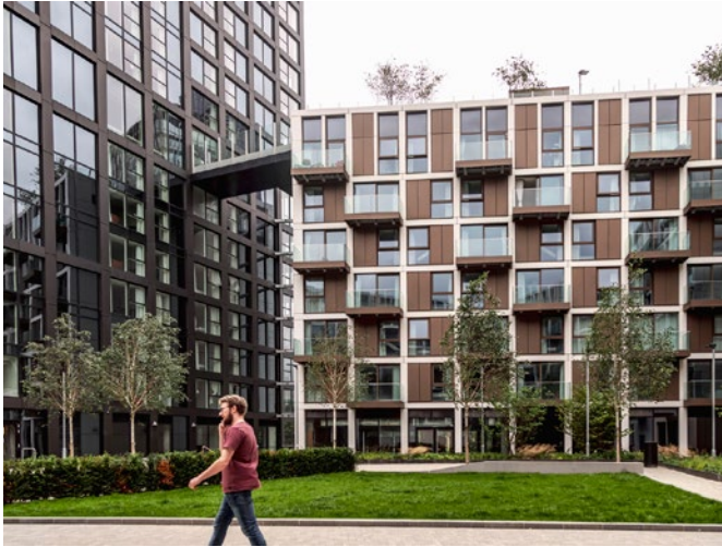
Angel Gardens, Manchester. High density urban apartments.
