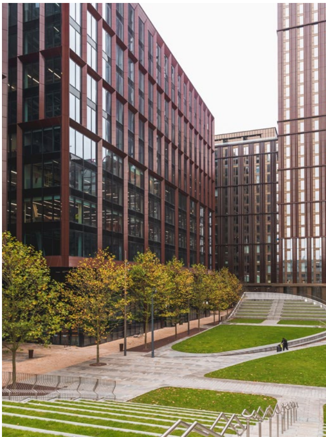
Circle Square, Manchester. High-rise, high-density living with generous park space
