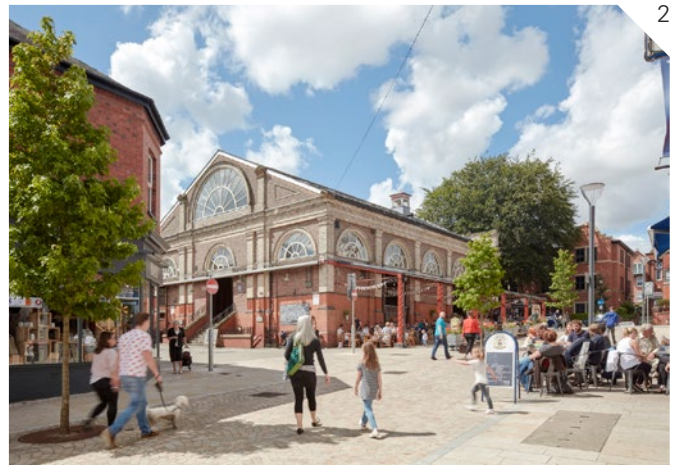
An example of a focal building with a balanced street - Altrincham Market, Shaw's Road, Altrincham
