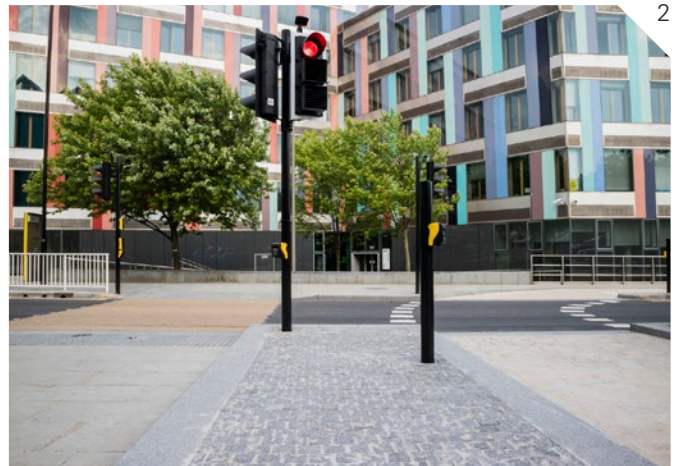
Example of a crossing with changes in surface treatment to delineate a change in priority for pedestrians and cyclists, and for vehicular traffic- Sheffield
