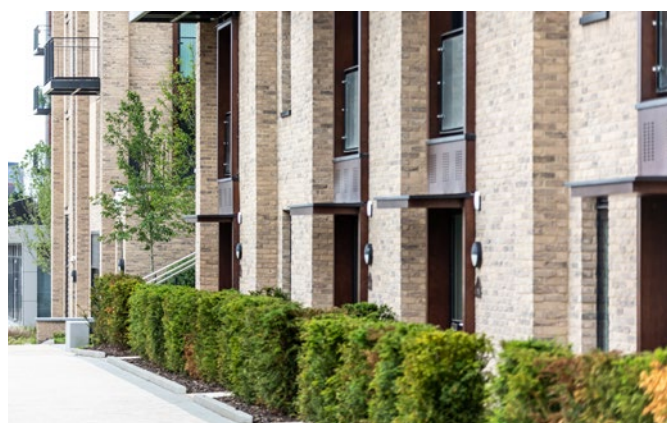
Duplexes providing regular doors onto the street at Middlewood Locks, Salford.
