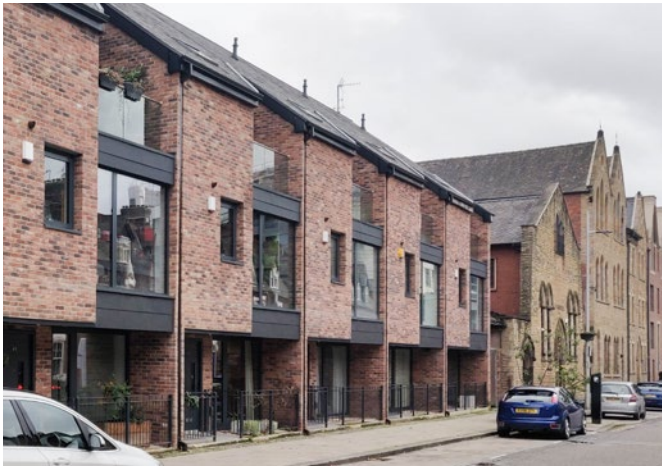
Mix of new and old. Townhouses in Ancoats, Manchester.
