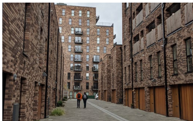
Maisonettes providing regular doors onto the street at Lockgate Mews, Manchester.
