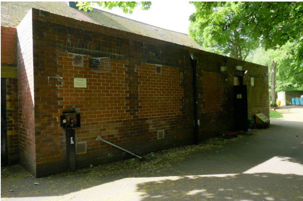
Photo 12 – Infilled windows and doors with different coloured bricks.
